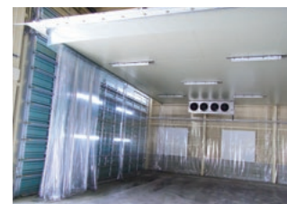
Example of soft vinyl curtain installation
