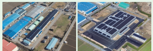
Achilles Corporation Shiga Factory No. 2
